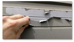
Sealants between precast concrete wall panels are deteriorating from age and UV exposure. Sealants are debonding from the concrete.
