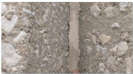
A site stone wall and gate secures the automotive parking area at the east elevation of the building. The site wall cap stones sealant and stone sealants are failed. Water is infiltrating the wall system. The metal gate accessing the secure parking area is corroding.
