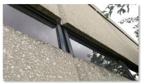
Larger, south elevation, windows are single pane and the gaskets are shrunken
