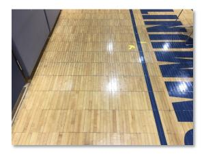
Finishes cracked and missing in several locations through-out building.
