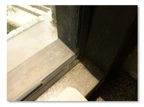
West elevation stair window system is allowing water into the building. This is causing corrosion of steel support member and CFMF.
