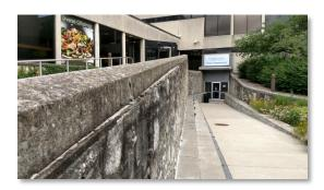
South elevation stair at gym: Slab-on-grade stair cracking and freeze-thaw deterioration.
