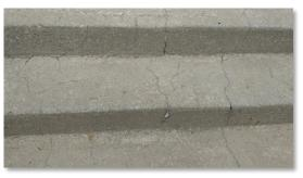
Southwest corner ramp: Loose rails and failed cove sealant at the stone wall causing deterioration of the stone/mortar.
