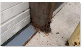
Wet seal repairs recommended around doors and associated glass panels. Paint peeling at garage doors, automotive bays.
