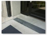
Water leak in Lower Level Room 007 below slab at recessed door and through abandon piping in wall.
