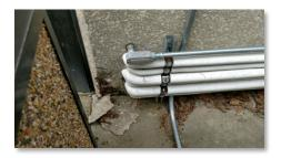
Paint coating at the walls surrounding the cooling tower is deteriorating from UV exposure.
