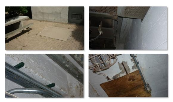
2. Slab and beams supporting the patio area outside the door to the southwest corner mechanical room are deteriorating from corrosion of embedded reinforcing steel. No or failed waterproofing may exist below the pavers.
