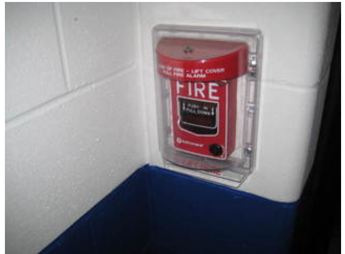
2002 Addition Fire Alarm System Manual Pull Station
