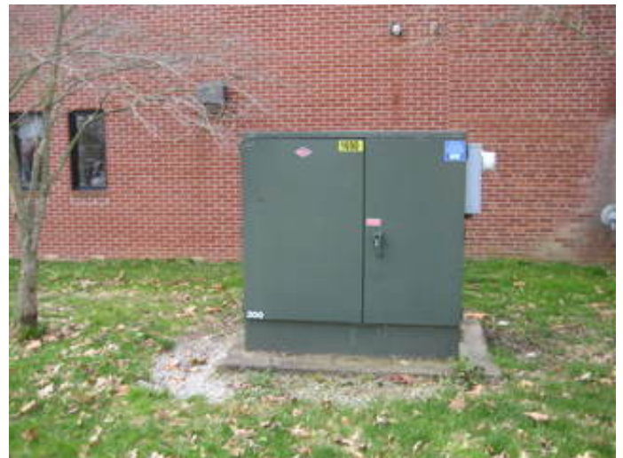
Pad Mounted Transformer
