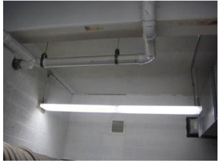
Sanitary Waste Piping
