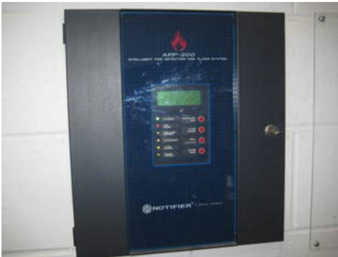
Fire Alarm System Control Panel
