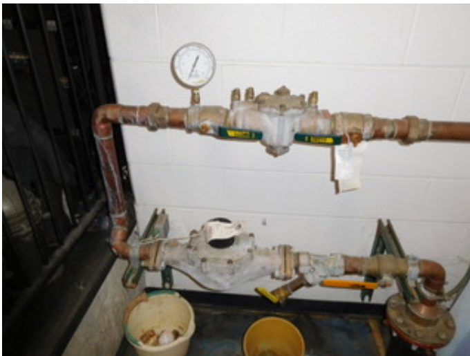
Incoming Domestic Water Service Backflow Preventer
