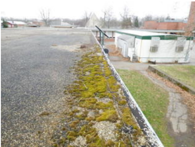
Built-Up Roof with Gravel Ballast
