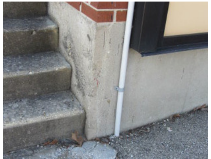
1957 Addition Exposed Concrete Foundation
