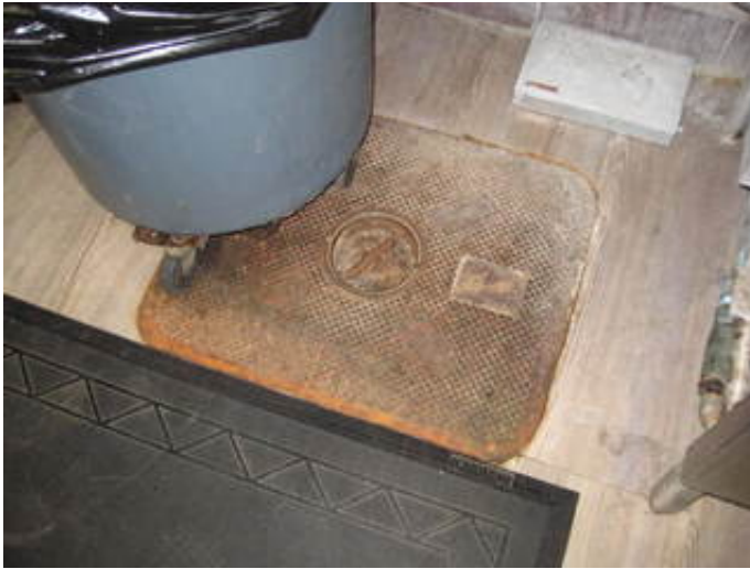
Kitchen Grease Trap Interceptor
