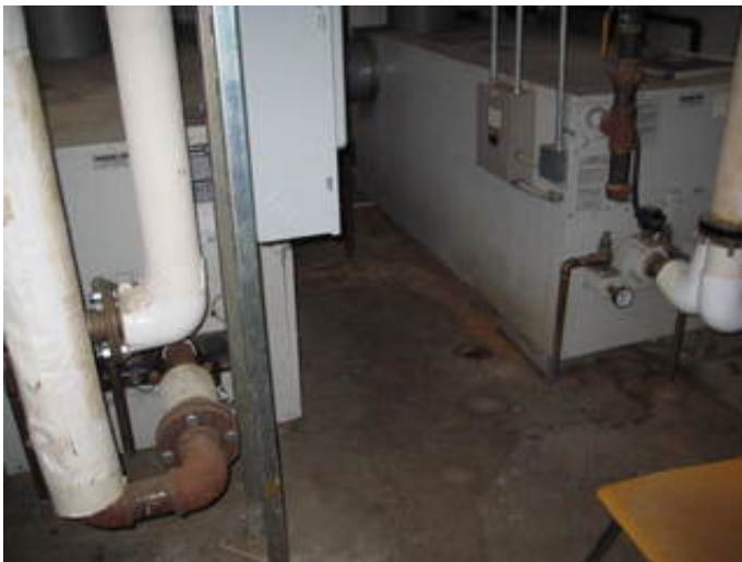
Natural Gas Fired Heated Water Boilers
