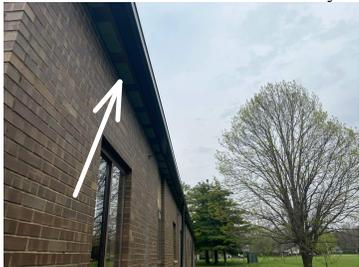
8. Shoe Boxes Exterior Surface: Brick(FAQ-Exterior) >>> Vent missing louver or cover (allowing air infiltration, potential for animals to enter)
