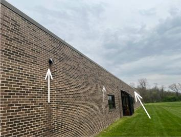
4. Shoe Boxes Exterior Caulking: Sealant >>> Joints around windows are not sealed (potential for water penetration)
