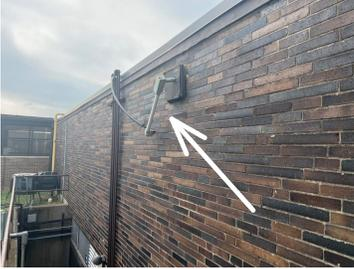
3. Rear Building Exterior Surface: Brick(FAQ-Exterior) >>> Roof scuppers emptying water down the wall which will cause problems with the brick
