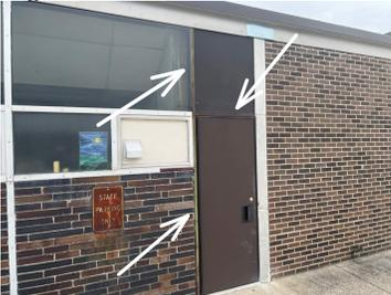
5. High Rise lower entrance area Exterior Windows: Aluminum Construction >>> Trim strips missing on stairwell windows
