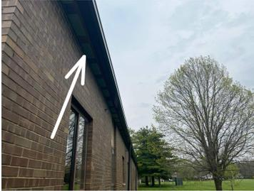
Surface: Brick(FAQ-Exterior) >>> Vent missing louver or cover (allowing air infiltration, potential for animals to enter)
