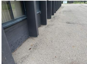
11. Surrounding Building Grounds Commercial Walkways: Concrete(FAQ-Sealants) >>> Deteriorated surface between pillars and blacktop
