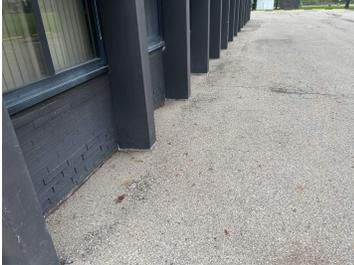
Walkways: Concrete(FAQ-Sealants) >>> Deteriorated surface between pillars and blacktop
