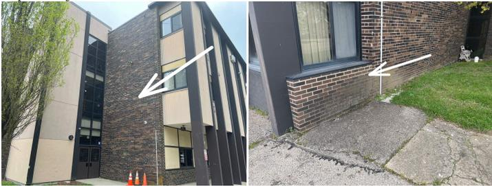
Surface: Exterior Insulated Finishing System (EIFS Stucco) (FAQ-Exterior) >>> Damaged areas on the lower panels: this is a poor choice of product for the lowest eight feet
