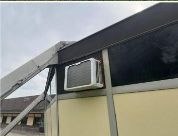
7. Shoe Boxes Exterior Surface: Metal Sheeting >>> Loose panels with water getting behind: Potential from moisture damage to substrate
