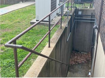
10. Surrounding Building Grounds Commercial Grading: Areas Need Attention >>> Grading has negative slope with potential for water pooling along foundation at the high rise stairwell (potential for damp problems in structure and premature foundation failure, any grading improvement to channel water away from the structure would be beneficial to foundation)
