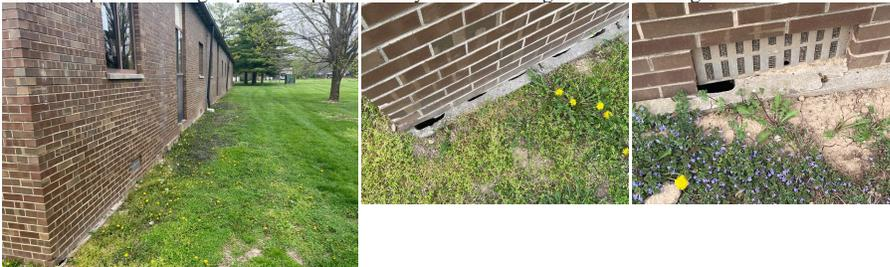
Caulking: Sealant >>> Joints around windows are not sealed (potential for water penetration)
