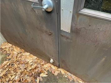
6. Music Room Exterior Surface: Transite Panels (possible asbestos content) >>> Four large panels damaged needing replacement
