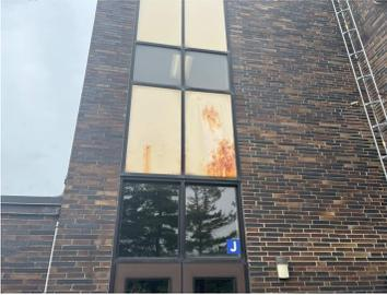
2. High Rise lower entrance area Exterior Surface: Brick(FAQ-Exterior) >>> End wall by the stair well may still not be secured to the buildings framing as required
