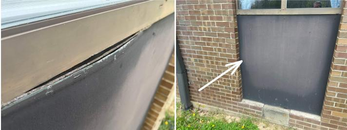
Foundation: Concrete Block Construction >>> Not matched up with the brick walls allowing for water to runoff the brick into the cavity and possibly into the crawlspace: flashing required: Approximately 3/4 of the length of the building
