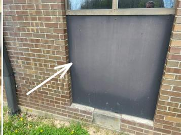
8. Shoe Boxes Exterior Foundation: Concrete Block Construction >>> Not matched up with the brick walls allowing for water to runoff the brick into the cavity and possibly into the crawlspace: flashing required: Approximately 3/4 of the length of the building
