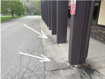
Stairwell Drain: Surface Type >>> Blocked by debris ( potential for flooding)
