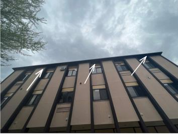
3. High Rise lower entrance area Exterior Surface: Galvanized Panels >>> Modified panel(s) where AC units were removed (allowing moisture intrusion, possible concealed damage to substrate)
