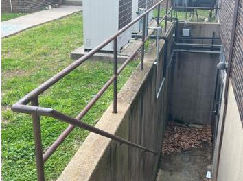
Grading: Areas Need Attention >>> Grading has negative slope with potential for water pooling along foundation at the high rise stairwell (potential for damp problems in structure and premature foundation failure, any grading improvement to channel water away from the structure would be beneficial to foundation)
