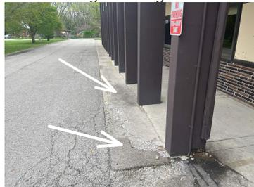
12. Surrounding Building Grounds Commercial Stairwell Drain: Surface Type >>> Blocked by debris ( potential for flooding)
