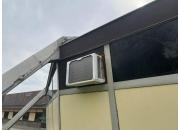
7. Shoe Boxes Exterior Surface: Metal Sheeting >>> Loose panels with water getting behind: Potential from moisture damage to substrate
