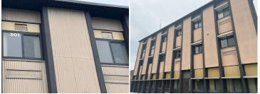
4. High Rise lower entrance area Exterior Trim: Aluminum >>> Missing (water damage possible) at door beside 112
