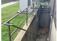
10. Surrounding Building Grounds Commercial Grading: Areas Need Attention >>> Grading has negative slope with potential for water pooling along foundation at the high rise stairwell (potential for damp problems in structure and premature foundation failure, any grading improvement to channel water away from the structure would be beneficial to foundation)
