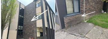
Surface: Exterior Insulated Finishing System (EIFS Stucco) (FAQ-Exterior) >>> Damaged areas on the lower panels: this is a poor choice of product for the lowest eight feet
