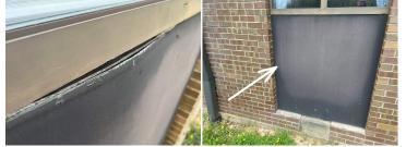
8. Shoe Boxes Exterior Foundation: Concrete Block Construction >>> Not matched up with the brick walls allowing for water to runoff the brick into the cavity and possibly into the crawlspace: flashing required: Approximately 3/4 of the length of the building\_\_\_\_\_
