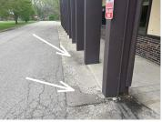
Stairwell Drain: Surface Type >>> Blocked by debris ( potential for flooding) Stairwell: Concrete Construction >>> Railing type does not meet today's standard for safety
