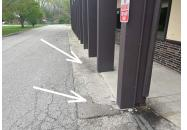
12. Surrounding Building Grounds Commercial Stairwell Drain: Surface Type >>> Blocked by debris (potential for flooding)
