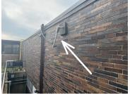
3. Rear Building Exterior Surface: Brick(FAQ-Exterior) >>> Roof scuppers emptying water down the wall which will cause problems with the brick
