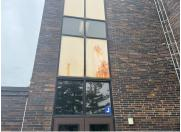
2. High Rise lower entrance area Exterior Surface: Brick(FAQ-Exterior) >>> End wall by the stair well may still not be secured to the buildings framing as required
