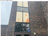
Surface: Brick(FAQ-Exterior) >>> End wall by the stair well may still not be secured to the buildings framing as required What appears to be a loadbearing steel plate outside window 117 supports the brick is failing Roof rain water pouring down the side of building close to door D : may affect foundation overtime Expansion joint not sealed below window front left corner
