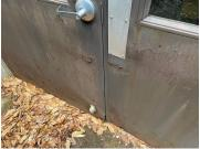
6. Music Room Exterior Surface: Transite Panels (possible asbestos content) >>> Four large panels damaged needing replacement Makeshift installation of window air conditioners: heating and cooling of this building may need to be evaluated
