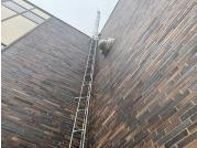
4. High Rise lower entrance area Exterior Caulking: Sealant >>> Joints failing (Potential for water intrusion) Particularly bad along the side with rooms 113 and 112
