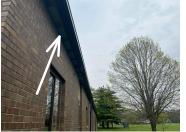
8. Shoe Boxes Exterior Surface: Brick(FAQ-Exterior) >>> Vent missing louver or cover (allowing air infiltration, potential for animals to enter) Poor location easy for animals to enter
