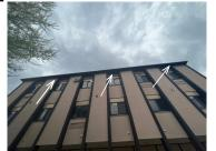
Surface: Galvanized Panels >>> Modified panel(s) where AC units were removed (allowing moisture intrusion, possible concealed damage to substrate) One wall air conditioner installed in the sheet-metal panel
