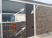
5. High Rise lower entrance area Exterior Windows: Aluminum Construction >>> Trim strips missing on stairwell windows A few window seals failing
