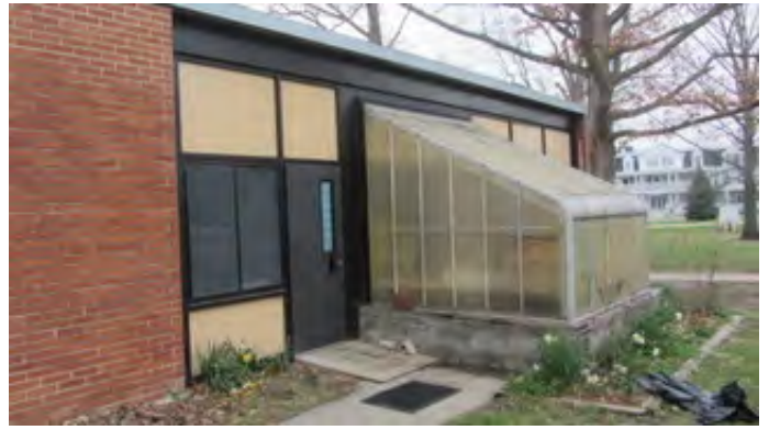
1957 Addition Typical Window System and Greenhouse
