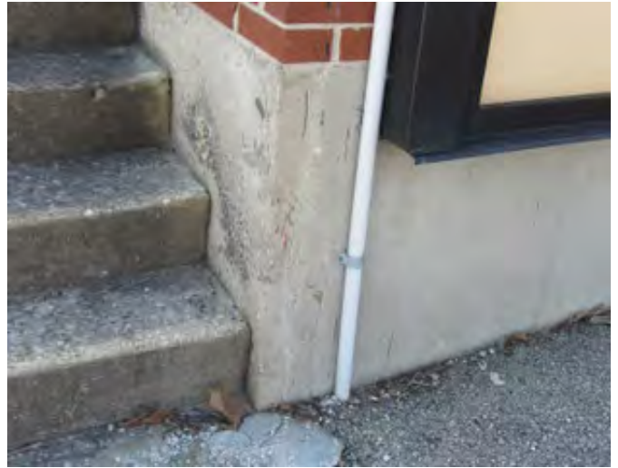
1957 Addition Exposed Concrete Foundation
