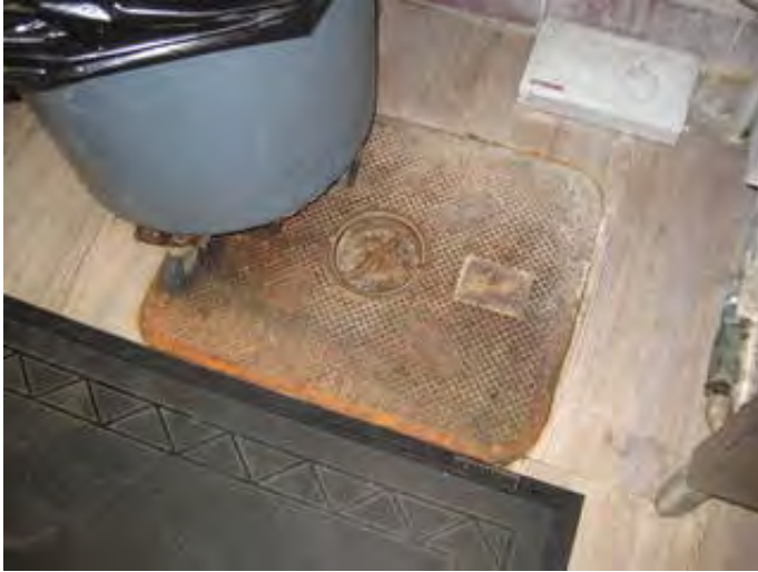
Kitchen Grease Trap Interceptor
