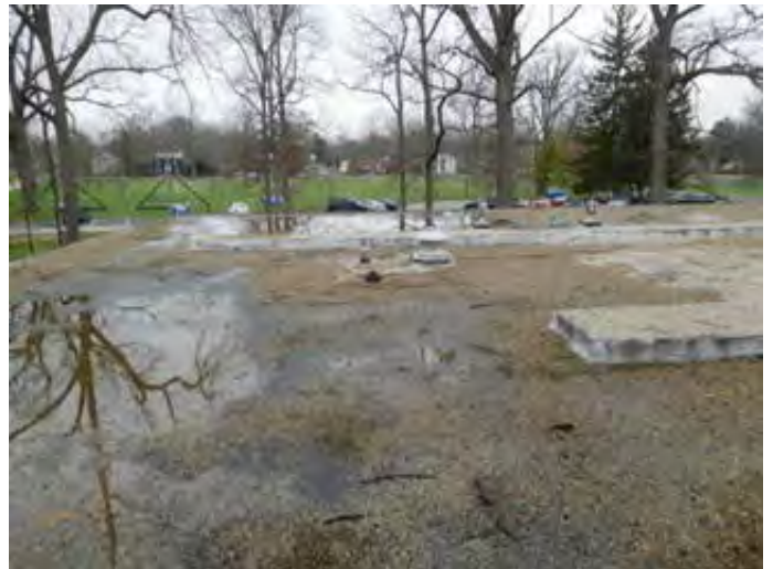
Built-Up Roof with Gravel Ballast
