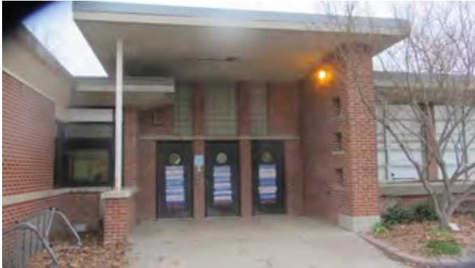
1952 Original Construction Main Entry Doors
