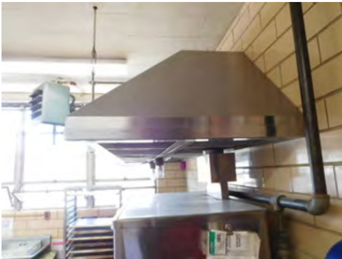
Existing kitchen hood in the Original Construction
