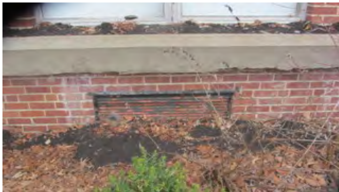
1952 Original Construction Window Sill and Unit Ventilator Opening
