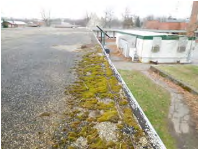
Built-Up Roof with Gravel Ballast
