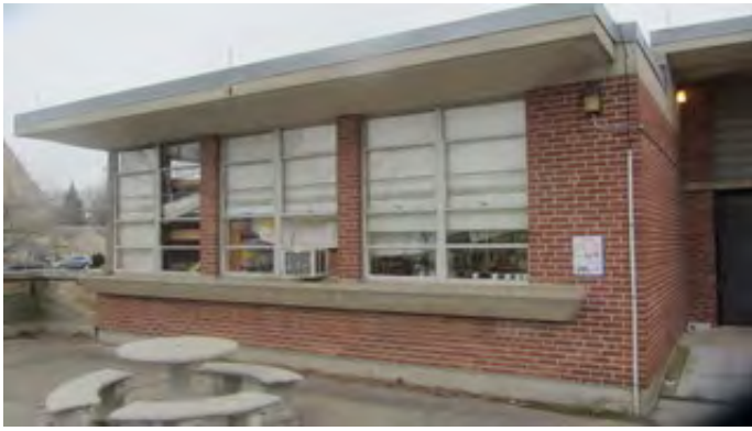
1952 Original Construction Typical Classroom Windows
