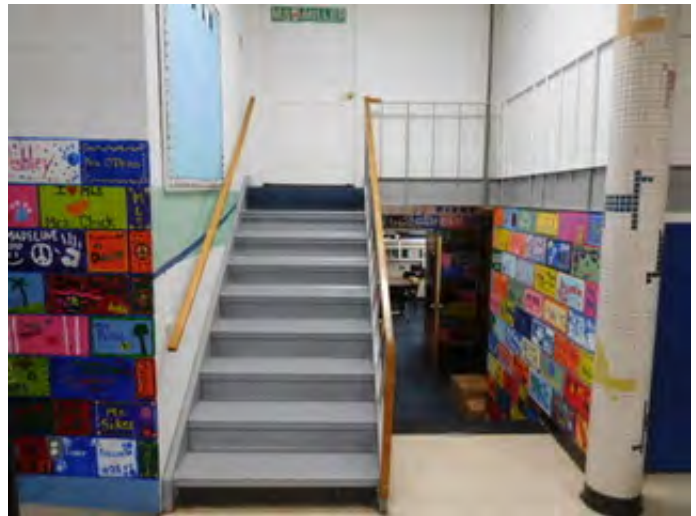
Stairs and handrail in the 1957 Addition
