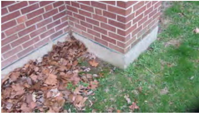
Typical 1952 Original Construction Exposed Foundation
