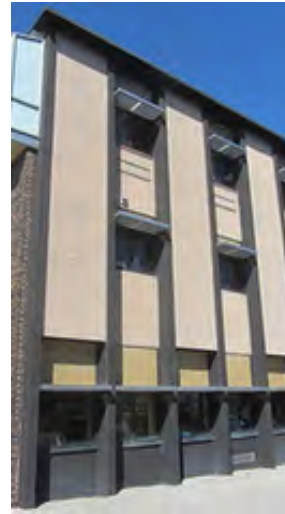
1963 Original Construction Three Story Structure
