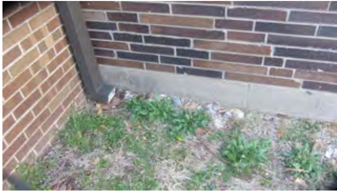
1963 Original Constructiton Exposed Foundation
