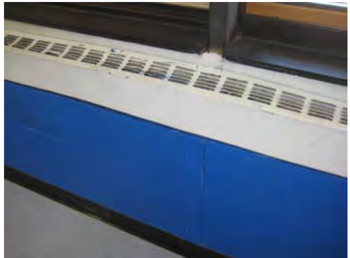
Heating Water Fin Tube Heater
