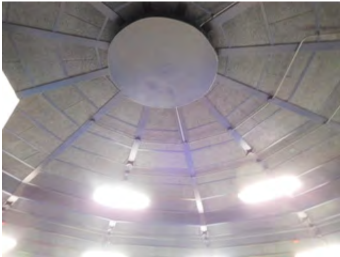
1963 Original Construction Music Room Roof Structure
