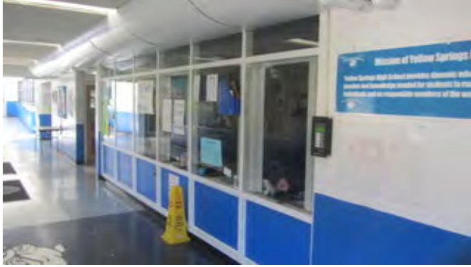
1963 Original Construction Interior Glazing
