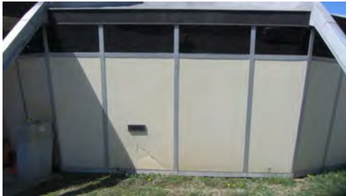
Insulated panels at 1963 Original Construction Music Room
