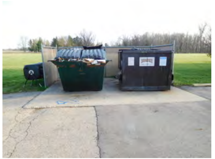
Concrete Dumpster Pad
