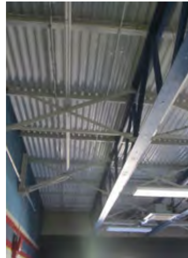
1963 Original Construction Student Dining Roof Structure
