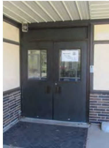
1963 Original Construction Main Entry Doors
