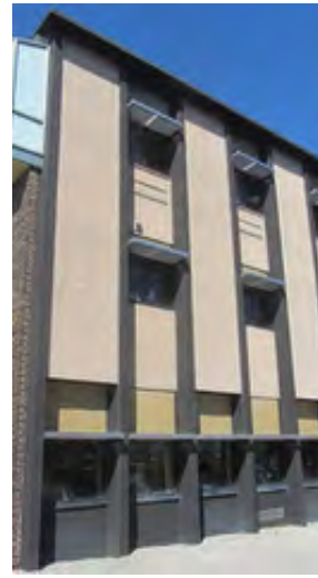
1963 Original Construction Classroom Windows
