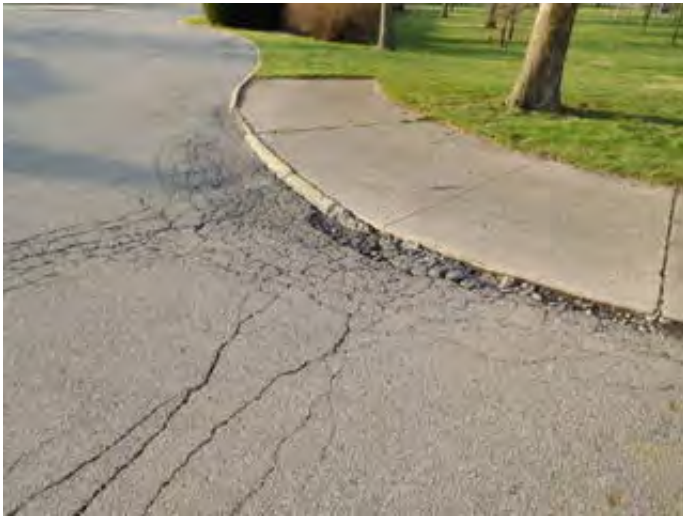
Asphalt, Curb, and Sidewalk Condition
