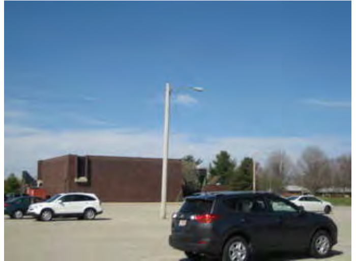
Pole Mounted HID High Pressure Sodium Light Fixture
